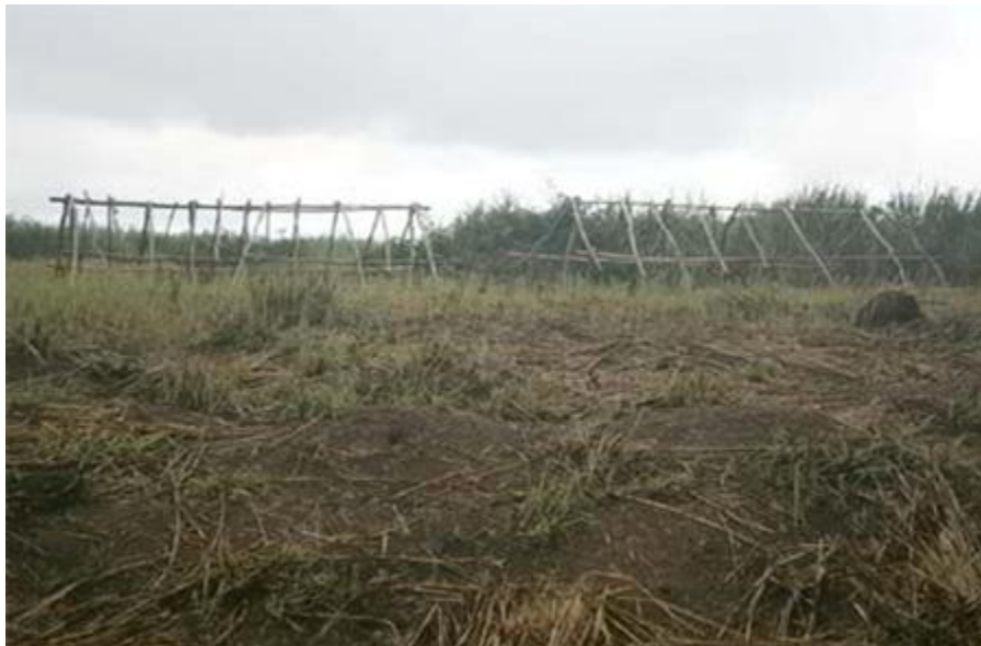
The school under construction
